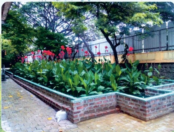
Vertical Flow Constructed Wetland (System B)
